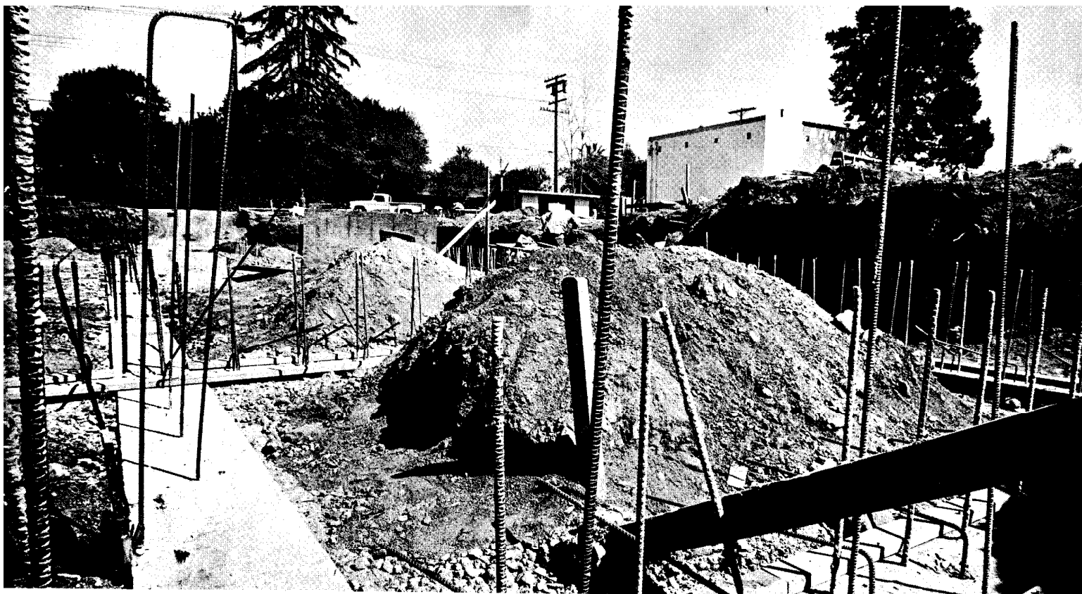
New gymnasium construction progresses rapidly.
