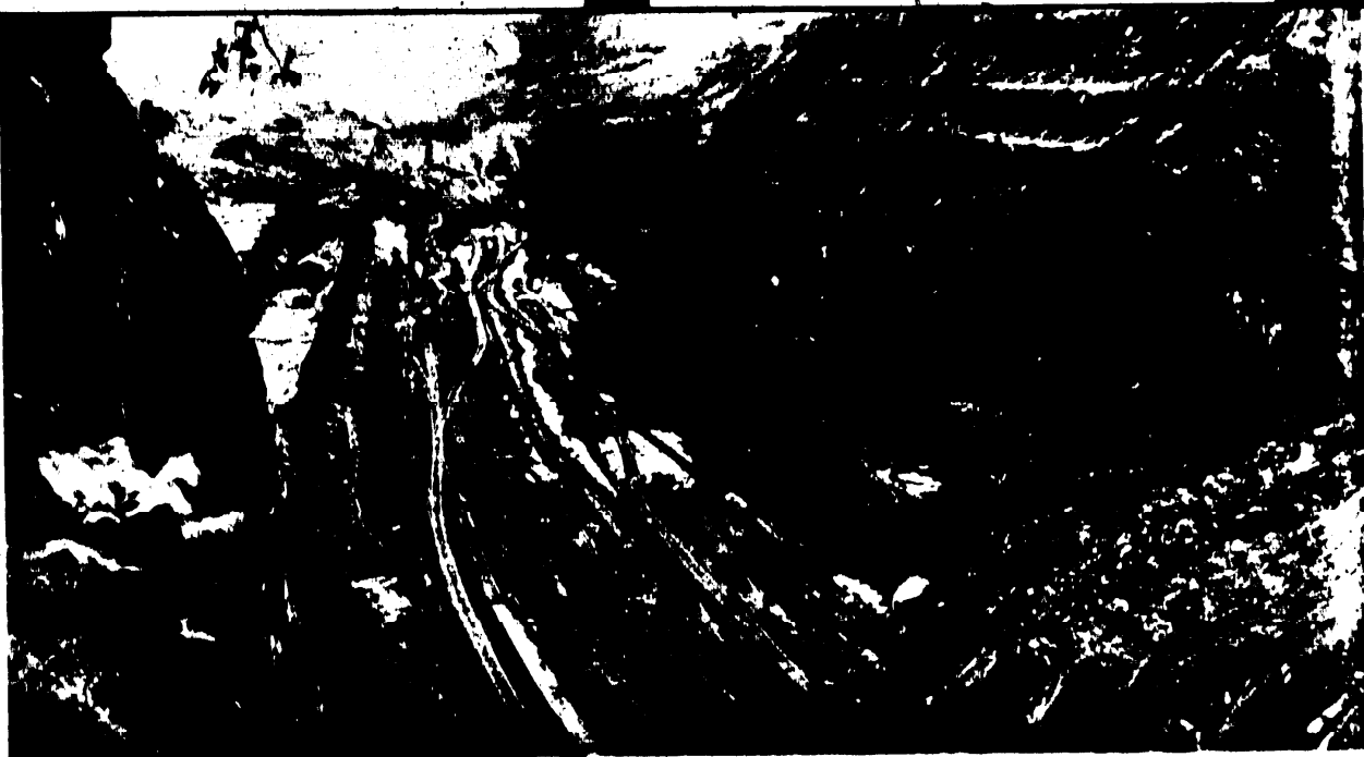
CUTTING THROUGH the Continental Divide on the Panamanian Isthmus in 1913. Landslides were a constant problem throughout Panama Canal construction. More than 200 million cubic yards of earth were excavated, one quarter of it slide material.
