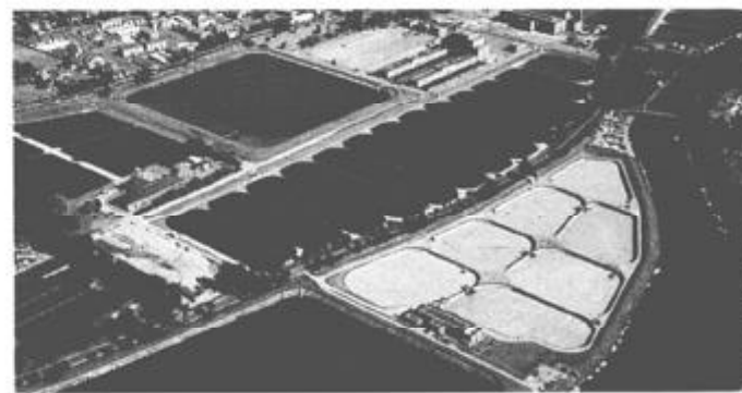
Water treatment facilities, Hampton, West London
